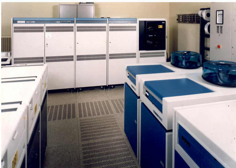
DEC VAX 11/780 at TNO (NL) (apparently running VAX/VMS)
